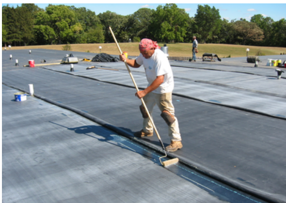
Applying EPDM with roller
