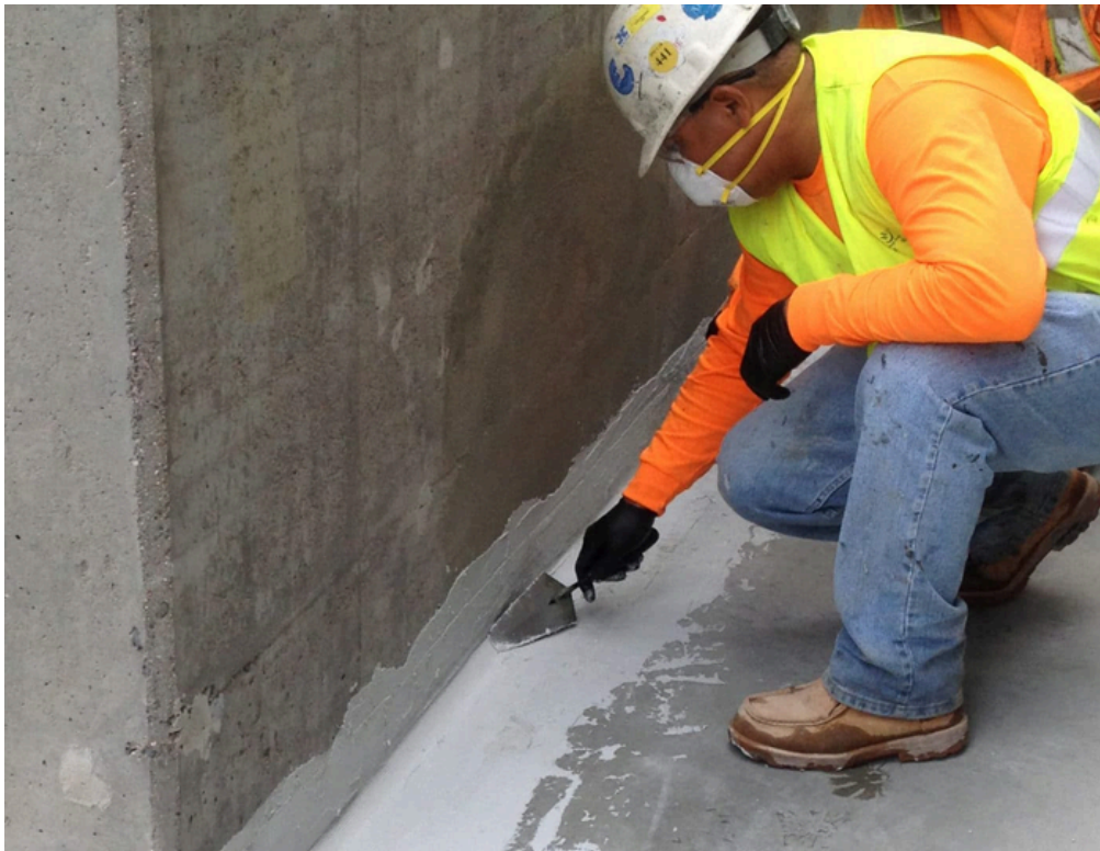
The application of cementitious waterproofing
