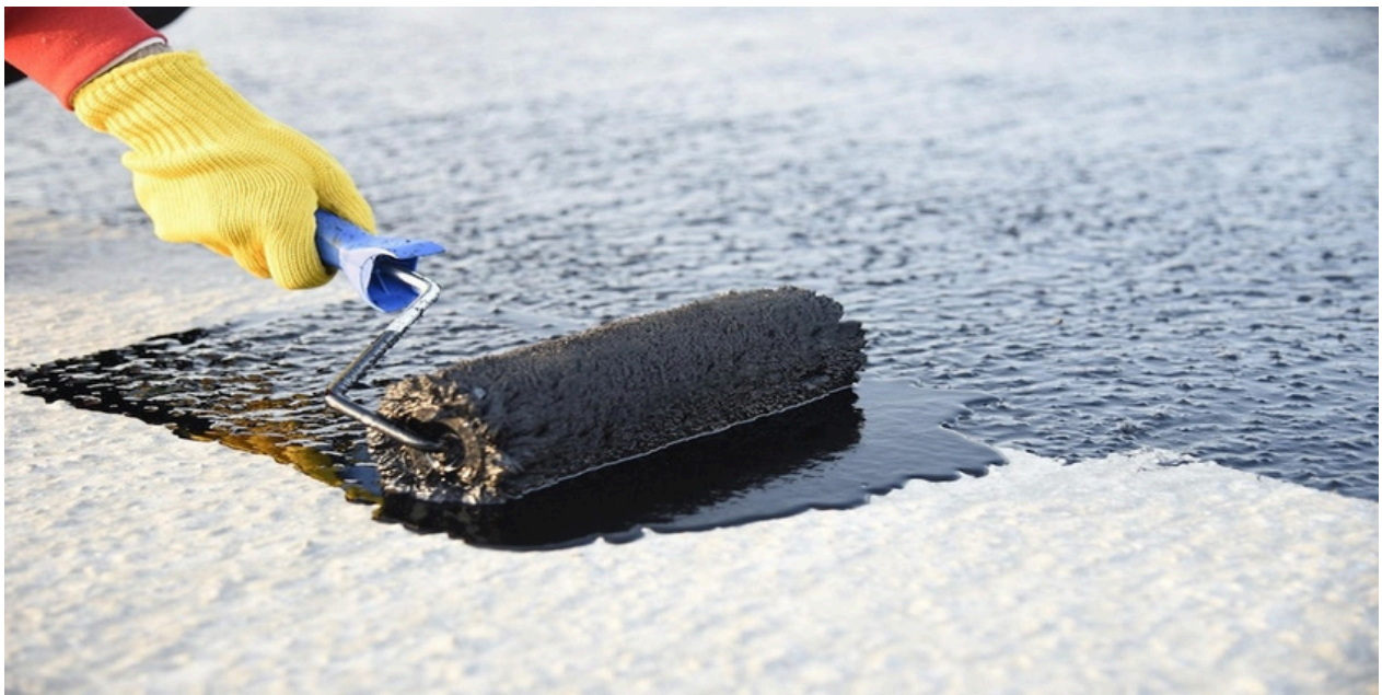
The application of Crystalline waterproofing .
