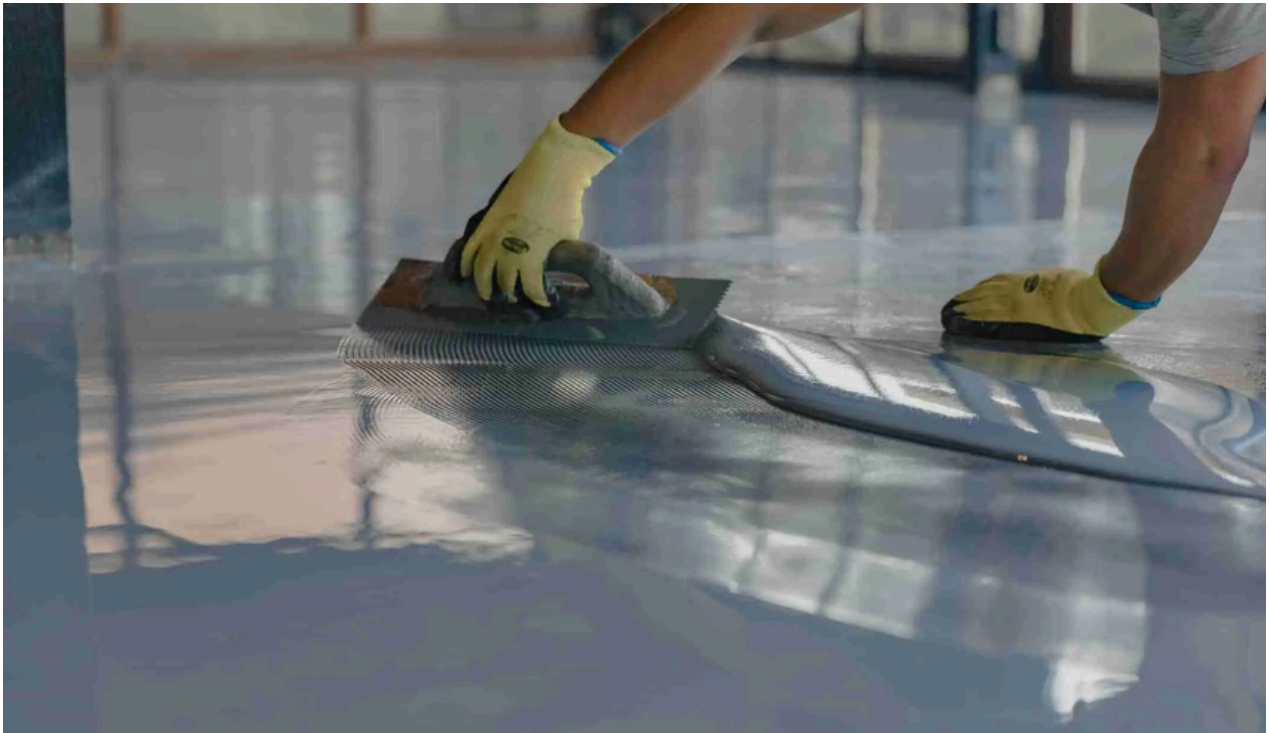
The application of epoxy painting works on the project site.
