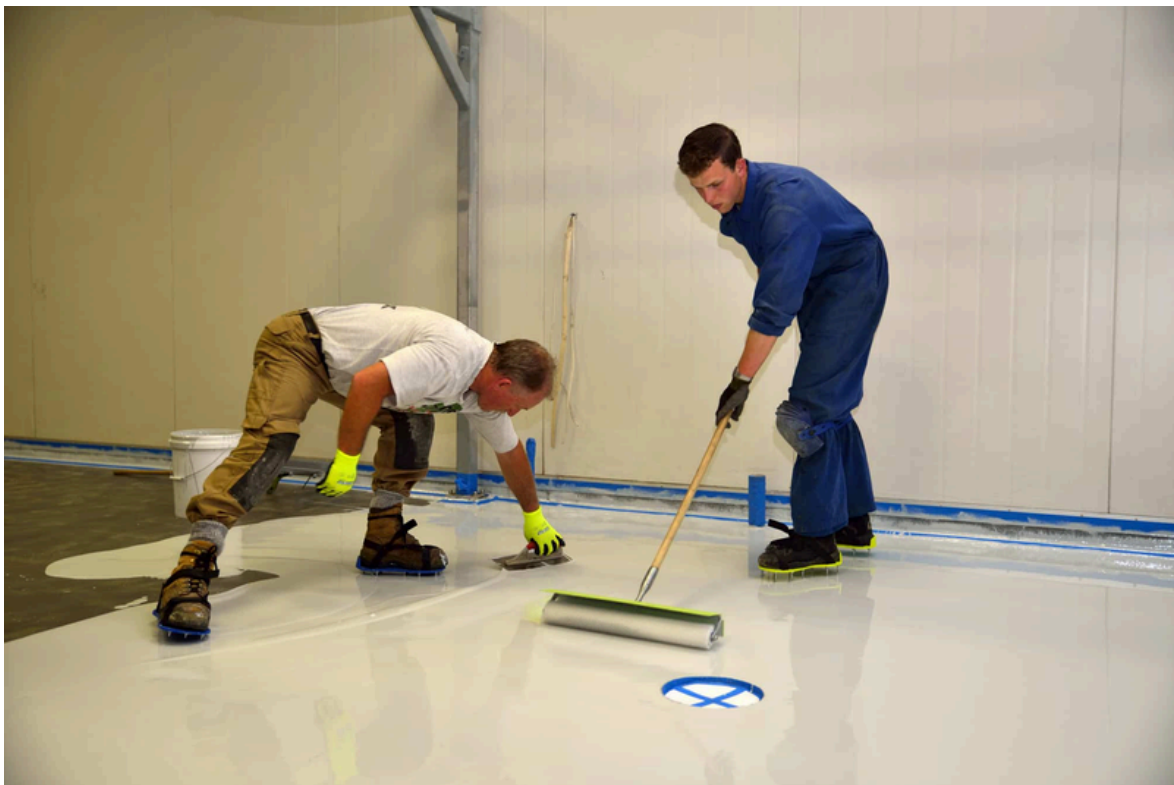
The application of non-toxic epoxy painting works on the project site.
