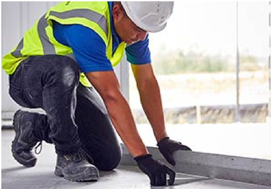
The asphalt base should be tested for planarity using a 10' straight edge
