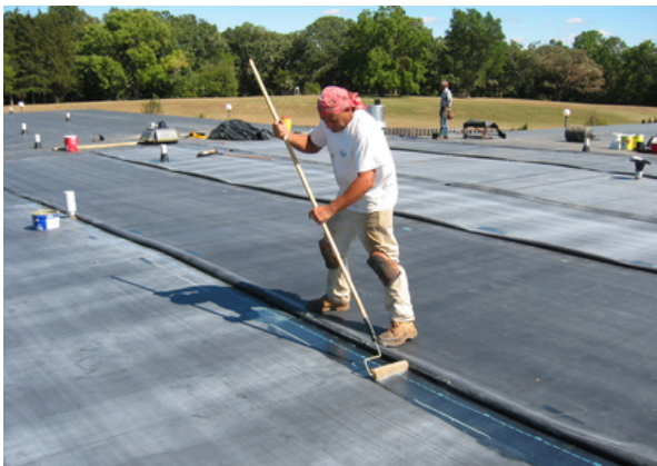
Applying EPDM with roller
