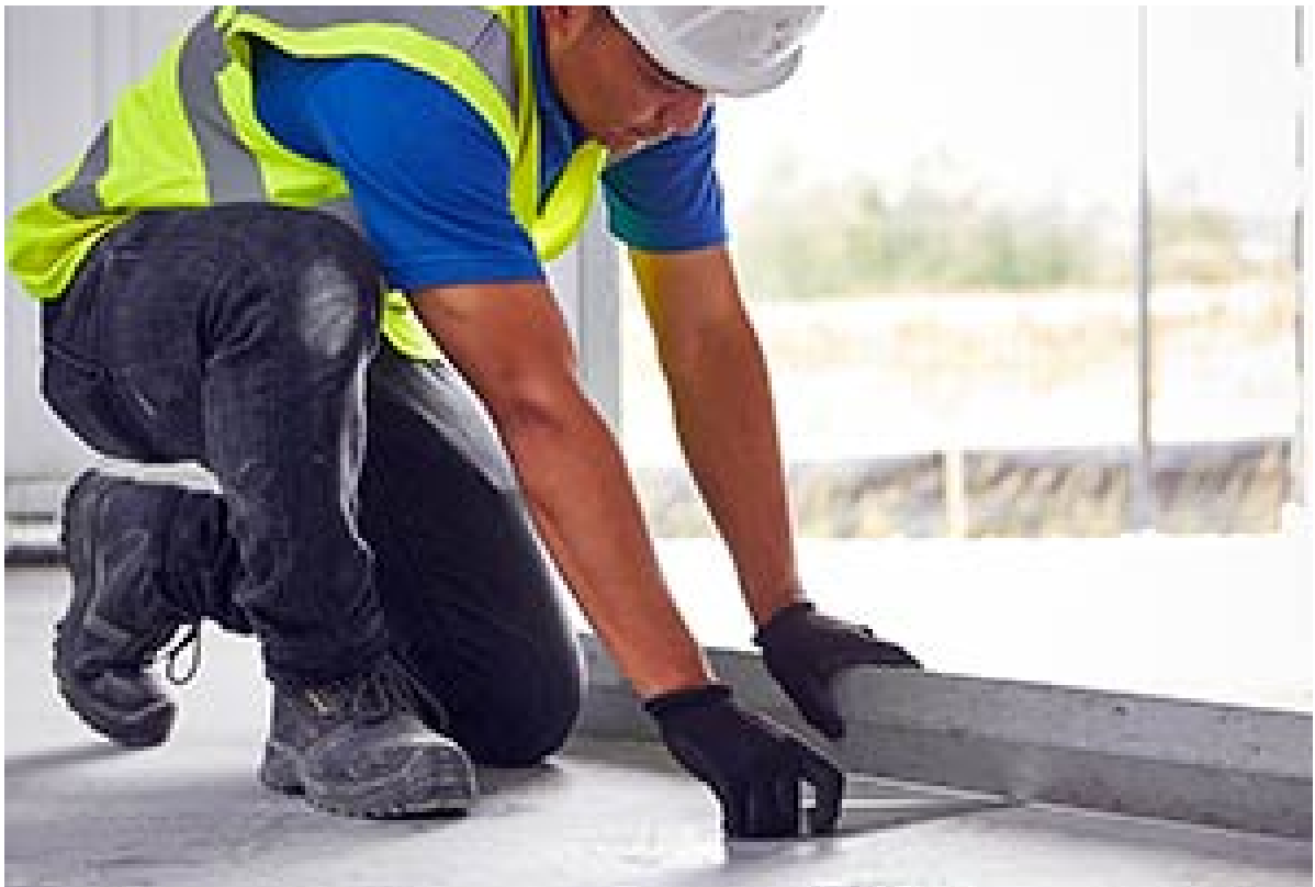
The asphalt base should be tested for planarity using a 10' straight edge
