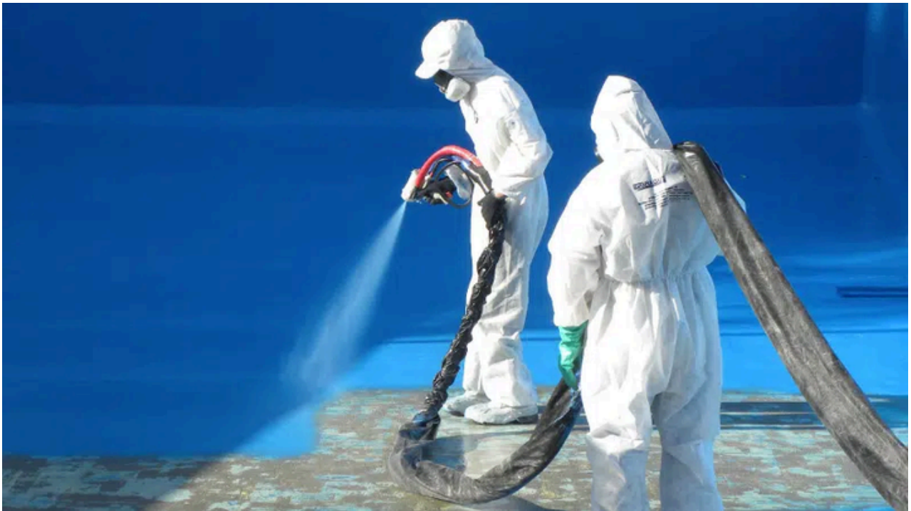
Application of sprayed polyurea membrane works.
